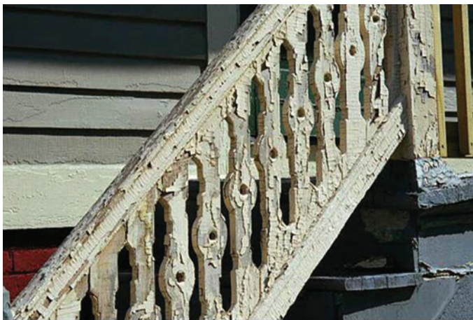
Outdoor stairs to a house featuring a banister with badly peeling paint.
